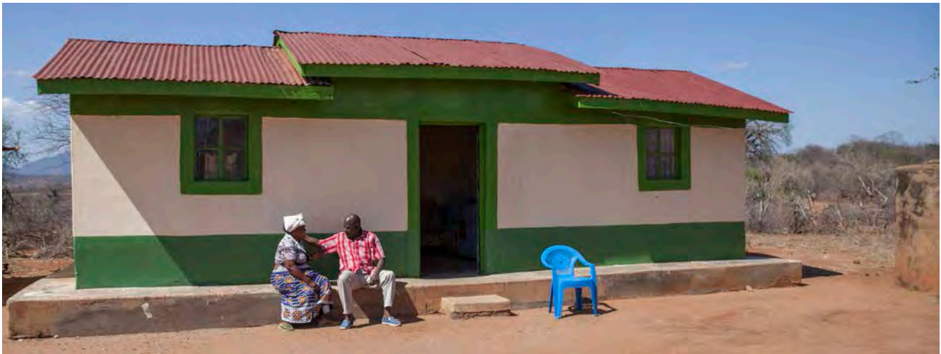
The Nyumba Smart Loan helped Annah and her husband complete their house, including installing a decorative steel door.
