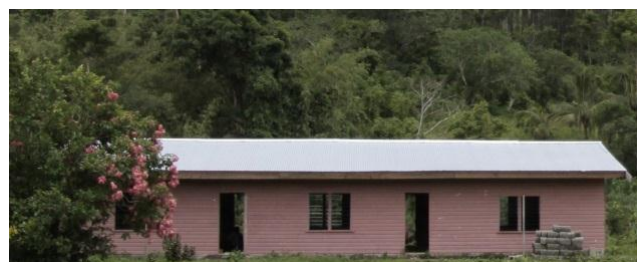
Figure 6: Village meeting house rebuilt after floods with funds from labour contracts
