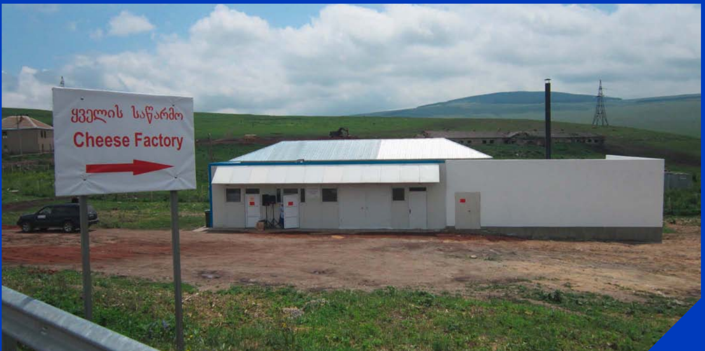
Dairy Products Company Tsezari, new facility, 2014 year, Sakdrioni village, Tsalka municipality
